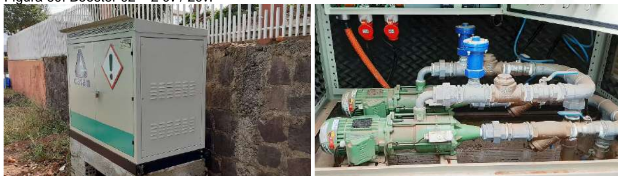
Figura 60: Booster 02 – 2 cv / 2cv.
